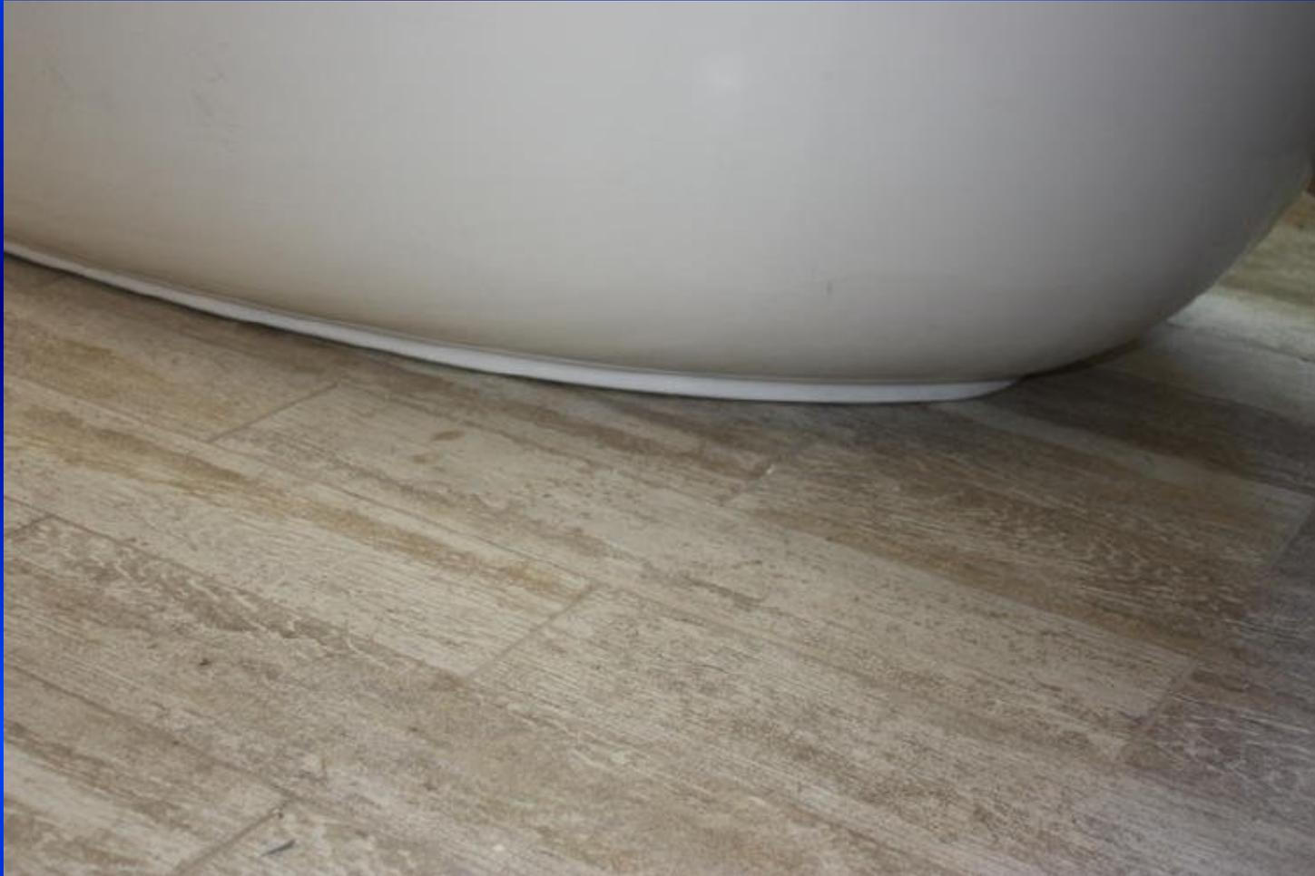
**The tub has been attached to the floor with silicone. This will ensure that there is no movement of the tub when it is without water.**
