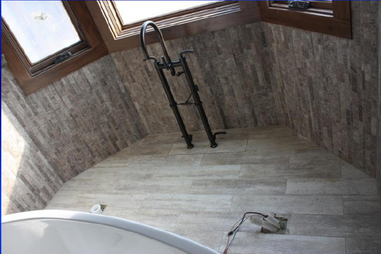
**This photograph illustrates a text book set-up. Note the pre-plumbed drain, piping and wiring. The wires were fed through a PVC pipe for protection as well as ease of installation.**
