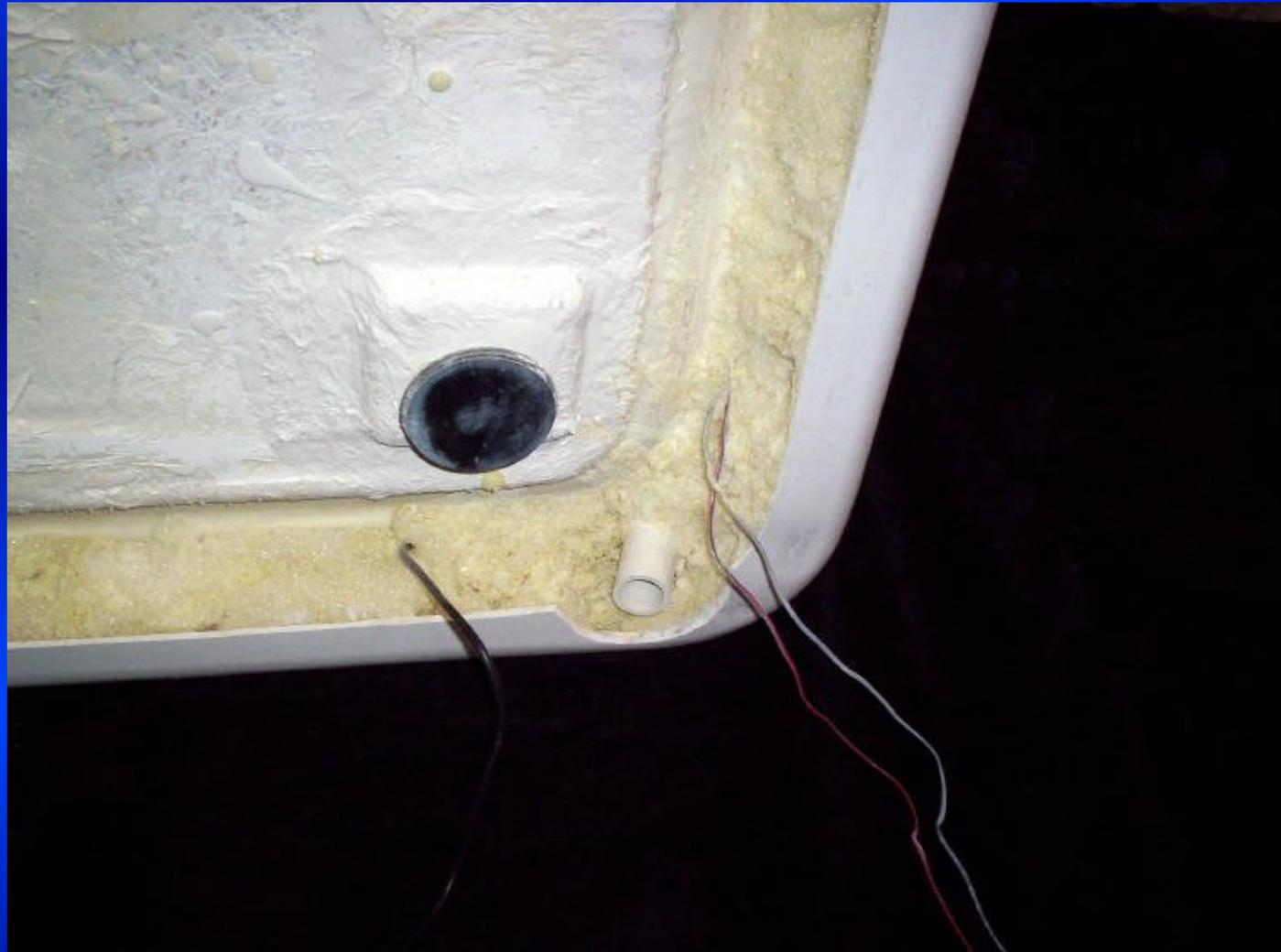
**Locate the blower connection and wiring under the tub. A cut out in the flooring will be necessary to allow the connection of the air piping as well as the wire routing.**
