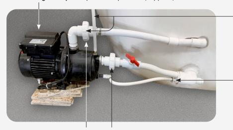
Air breather tubing with check valve must be straight up (you can zip-tie it to the union connection).
